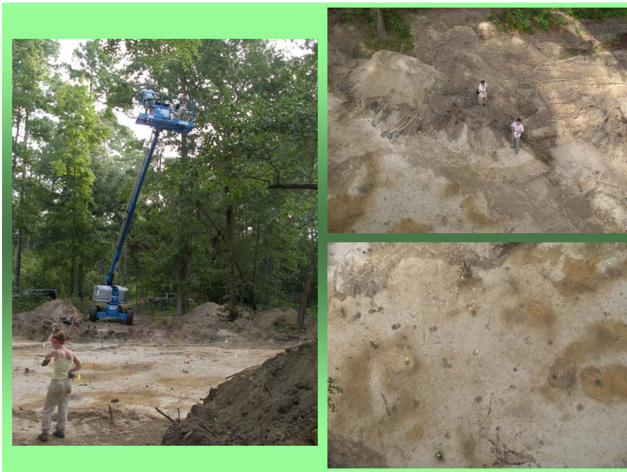
Figure 7. Clockwise from top left: a) use of a boom-lift to obtain a bird's eye view of the exposed excavation floor; b) archaeologists examining cultural features in the excavation floor; c) view from the boom-lift over the excavation floor.
